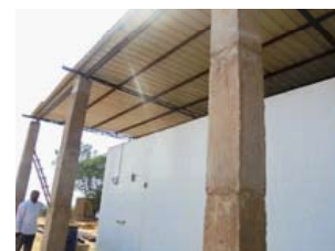
Cold storage unit (under construction)
